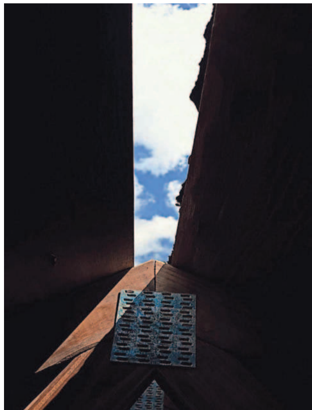
ABOVE: The Libby Road home of Jeffrey and Virginia Rapkin was heavily damaged by Hurricane Ian. The city of North Port has refused to allow FEMA to put a two-bedroom mobile home on their property because of a city ordinance that does not allow manufactured homes in single-family lots.
